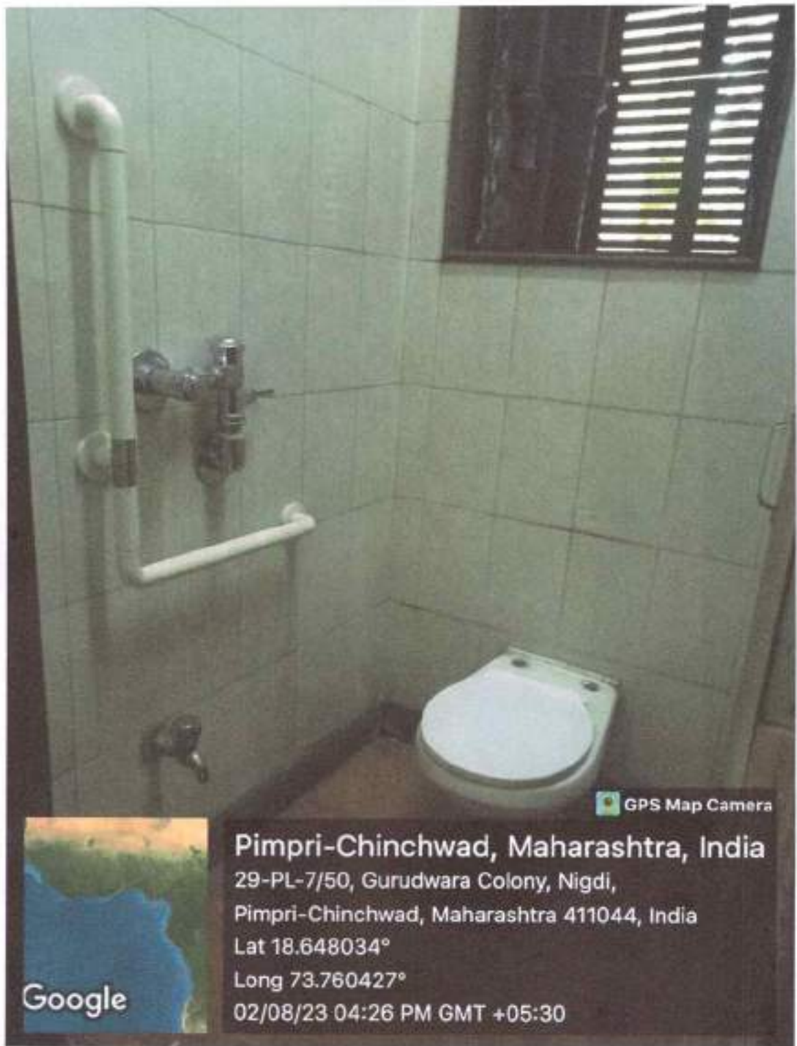
Geotagged Photograph of installation of grab bar at female toilet.
