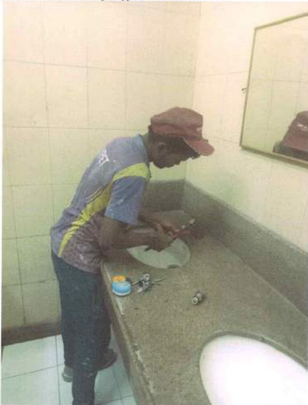
Installation performed by an expert in female toilet at college campus.
