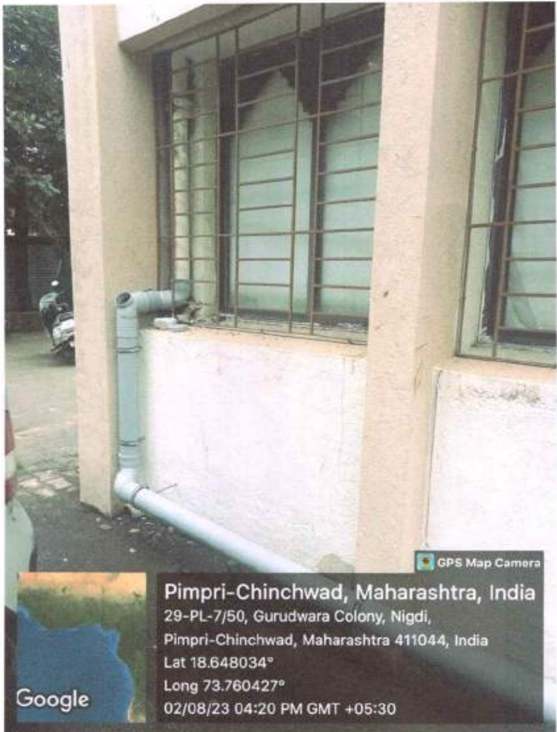
Geotagged picture of downpipe in rain water harvesting system at campus
