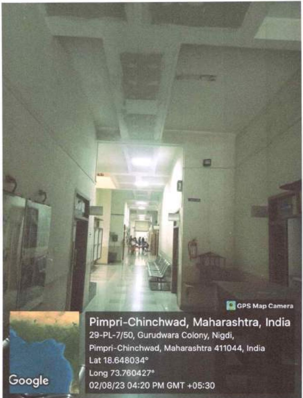
Installation of LED Tube in campus Corridor area.
