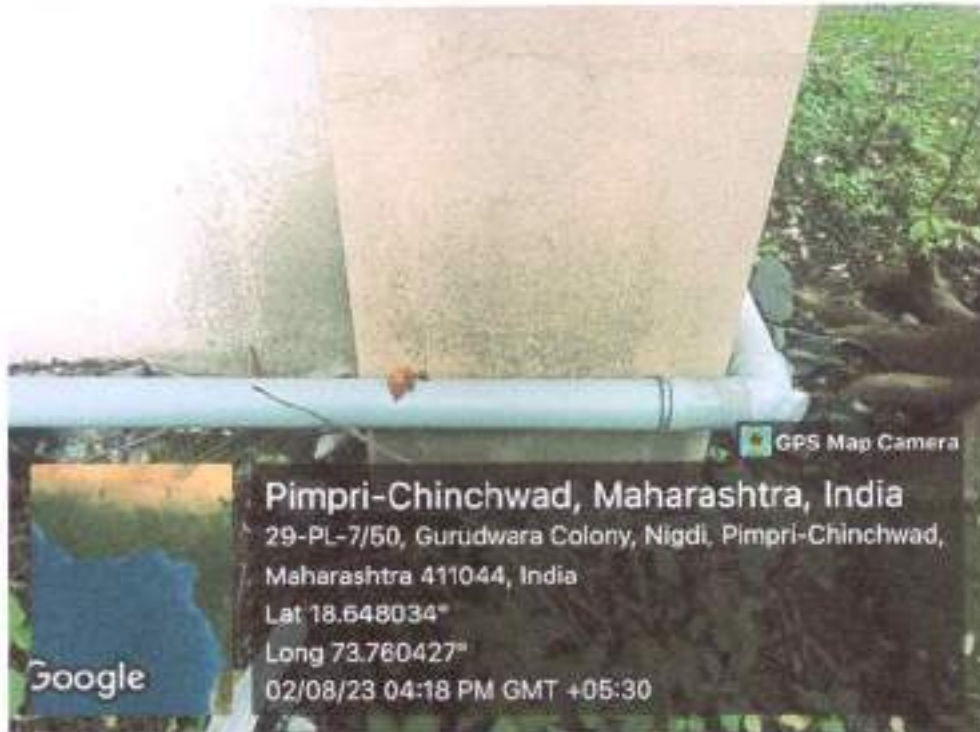
Geotagged photograph of downpipe second location.
