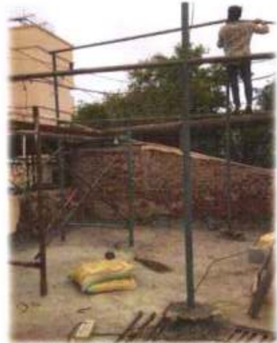
ROOFING FRAME OVER TOILET AREA
