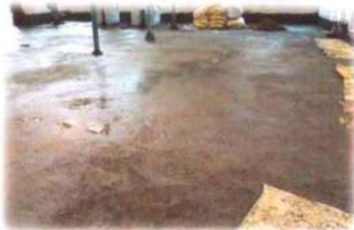
WATERPROOFING COAT OVER SLAB
