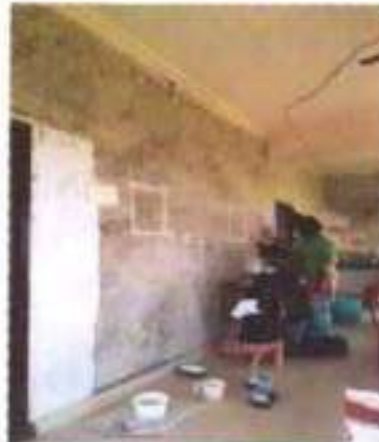
2. MARKING FOR LIME PLASTER
