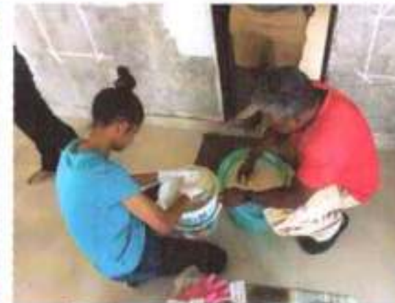
3. PREPARATION OF MIXTURE FOR PLASTERING. ( BEFORE APPLICATION POWDERED LIME SOAKED IN WATER OVERNIGHT )
