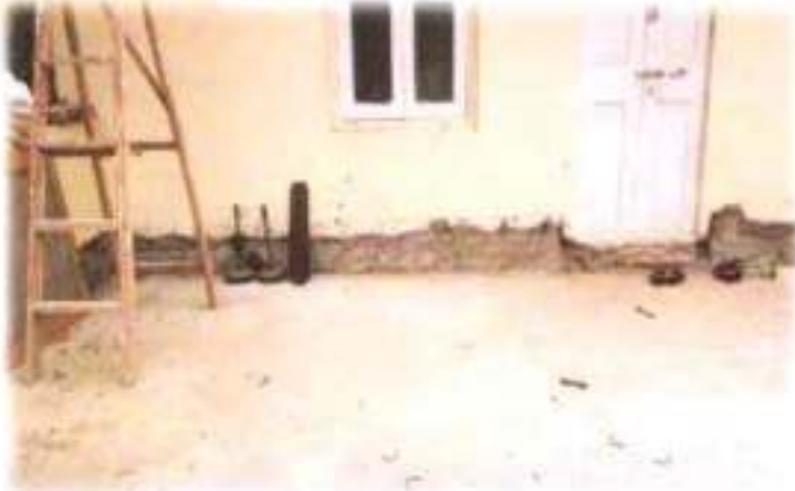
REMOVAL OF 11 TH LAYER OF PREVIOUS WATERPROOFING LAYER TILL SLAB
