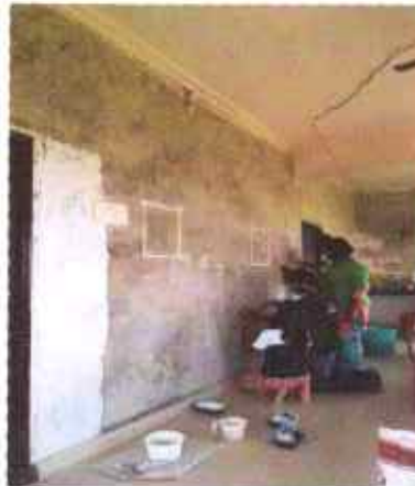
2. MARKING FOR LIME PLASTER
