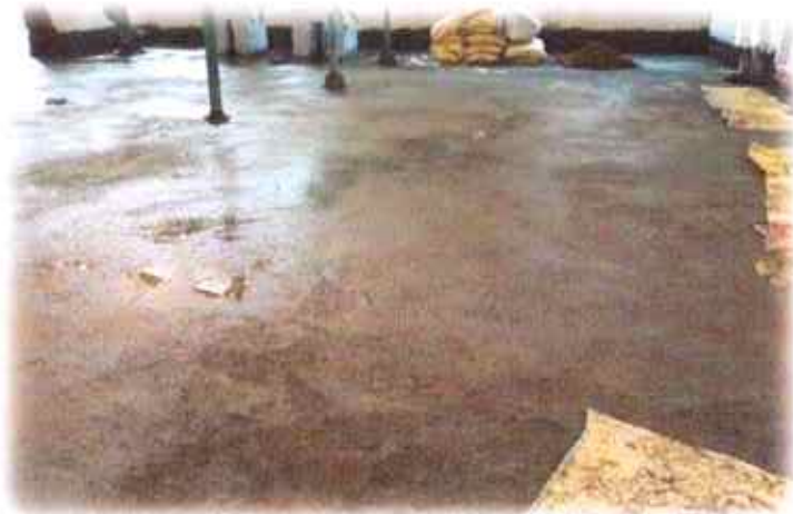
WATERPROOFING COAT OVER SLAB
