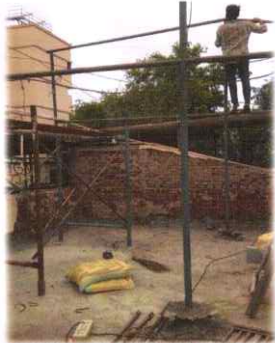
ROOFING FRAME OVER TOILET AREA
