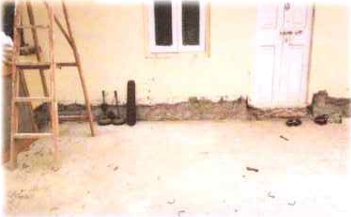
REMOVAL OF 11" LAYER OF PREVIOUS WATERPROOFING LAYER TILL SLAB
