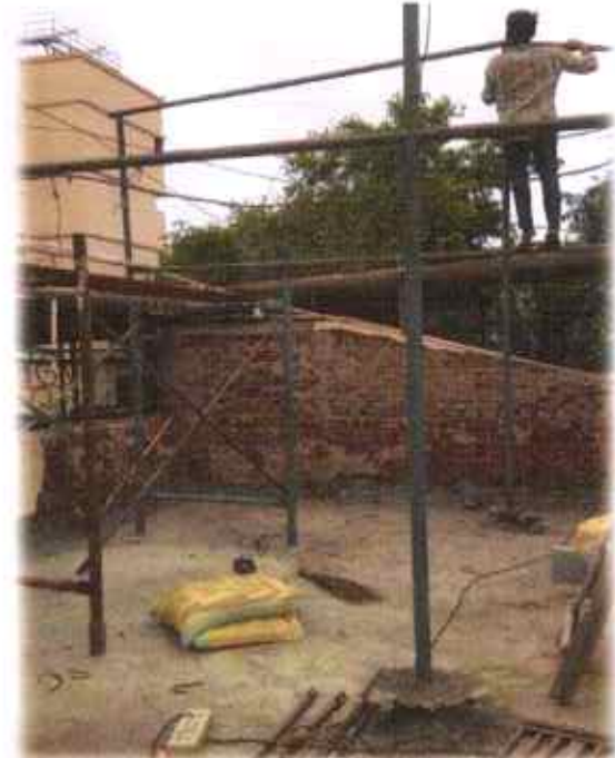
ROOFING FRAME OVER TOILET AREA
