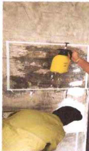
5. CURING OF SURFACE WITH WATER BEFORE APPLYING LIME PLASTER
