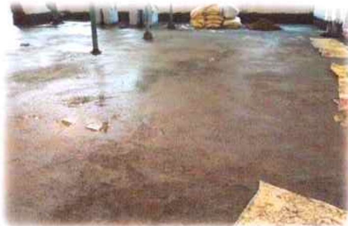
WATERPROOFING COAT OVER SLAB
