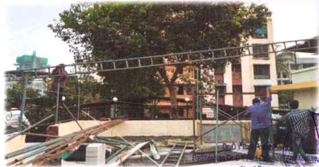
REMOVAL OF PREVIOUS ROOFING AND NEW FRAMEWORK FOR EXTENDED ROOFING
