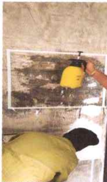
5. CURING OF SURFACE WITH WATER BEFORE APPLYING LIME PLASTER
