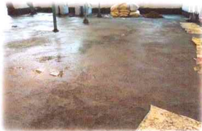
WATERPROOFING COAT OVER SLAB
