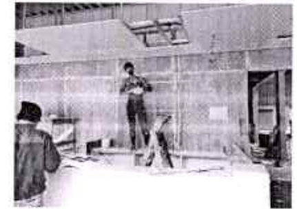
FALSE CEILING WORK
