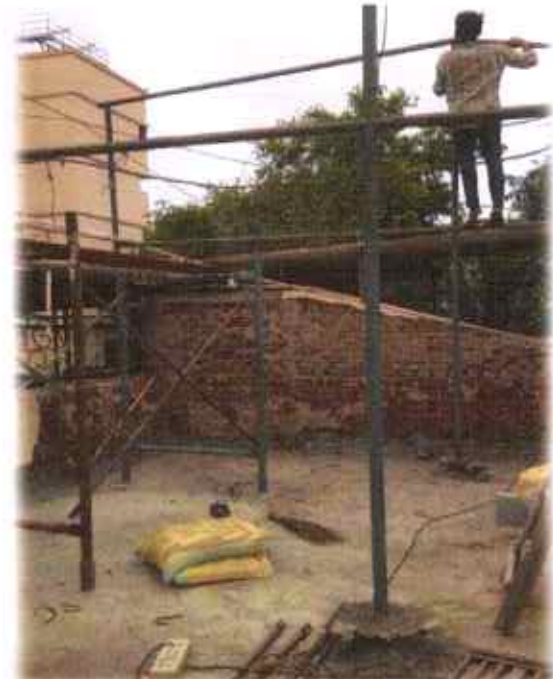
ROOFING FRAME OVER TOILET AREA
