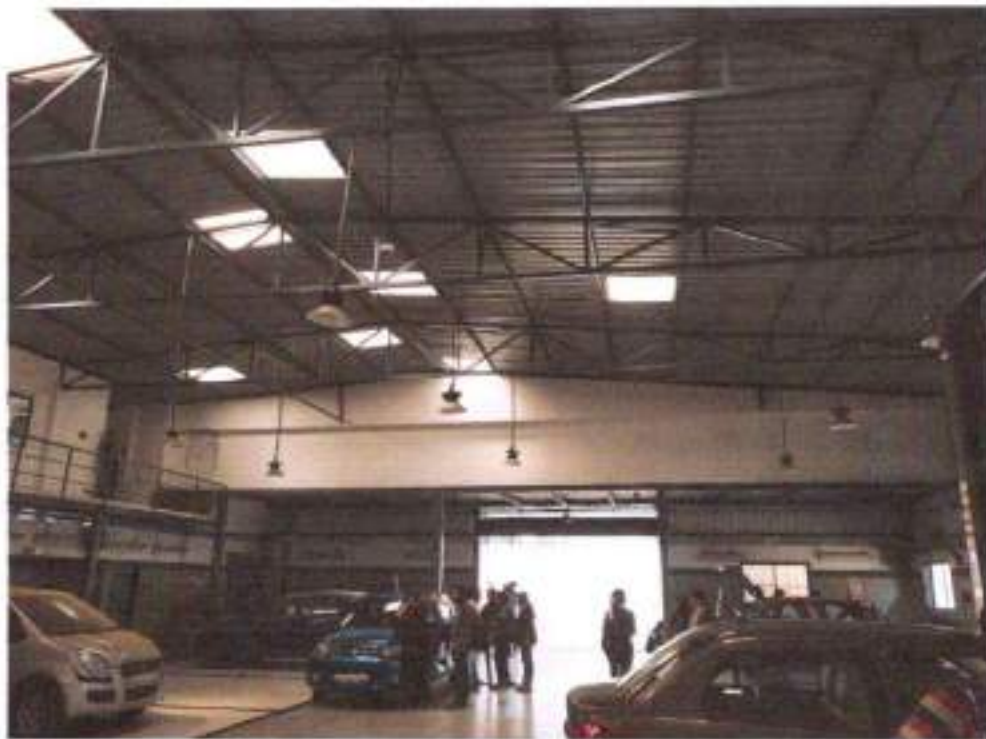
Students taking Photo and notes at Skoda Showroom for steel Structure
