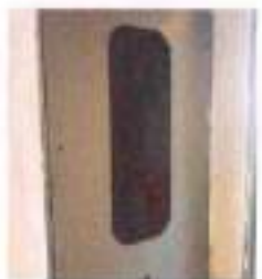
FIRE RATED DOOR FOR THE SHAFT TO BEAT FIRE FOR 2 HOURS
