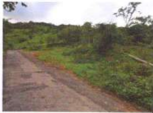
Approach road to the site
