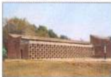
Sun breaker is provided at facade
