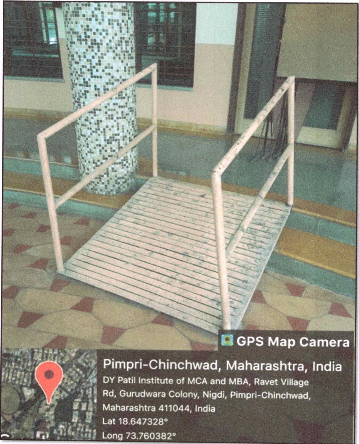
Ramp provision for in campus movement.
