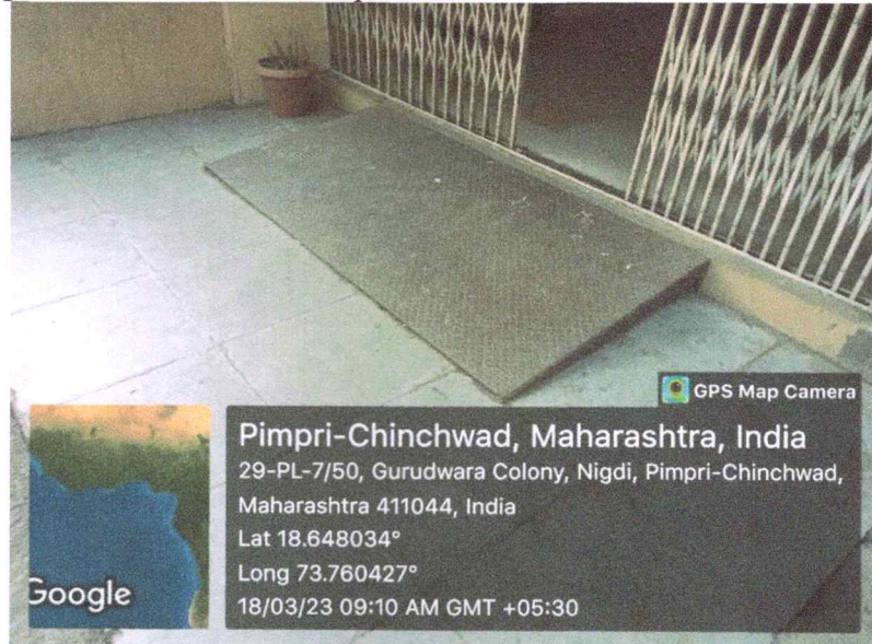
Cast iron ramp on entrance for disabled person
