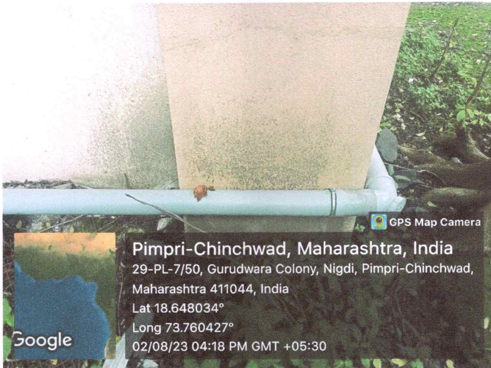
Geotagged photograph of downpipe second location.
