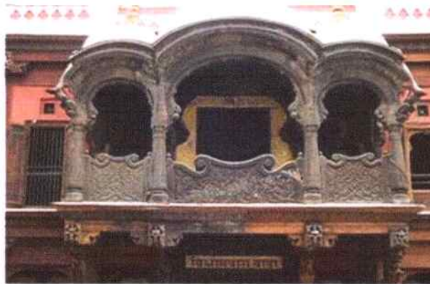
TIMBER BALCONY AT VISHRAMBAGHWADA
